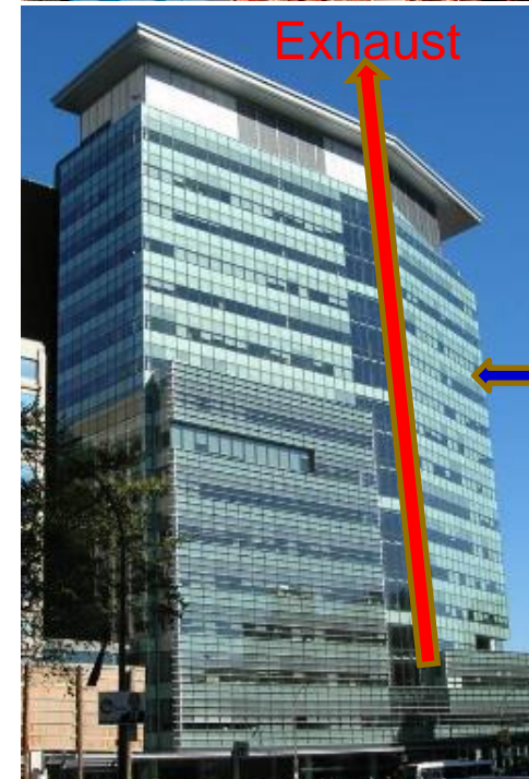
EV building hybrid ventilation system
